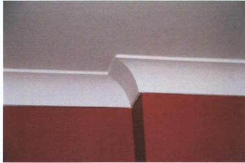
Plate 76: T-2 – Detail to coving to chimney breast
