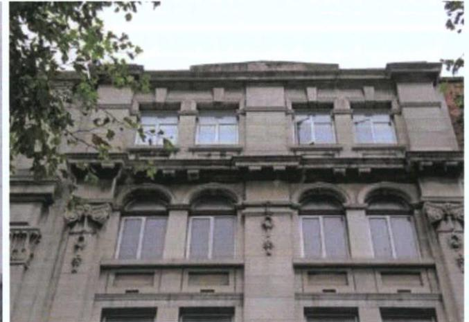
**Fig. 13** Pediment parapet featuring the inscription '1925'. Note timber transom and arched head on Level 3, and also Level 1.
