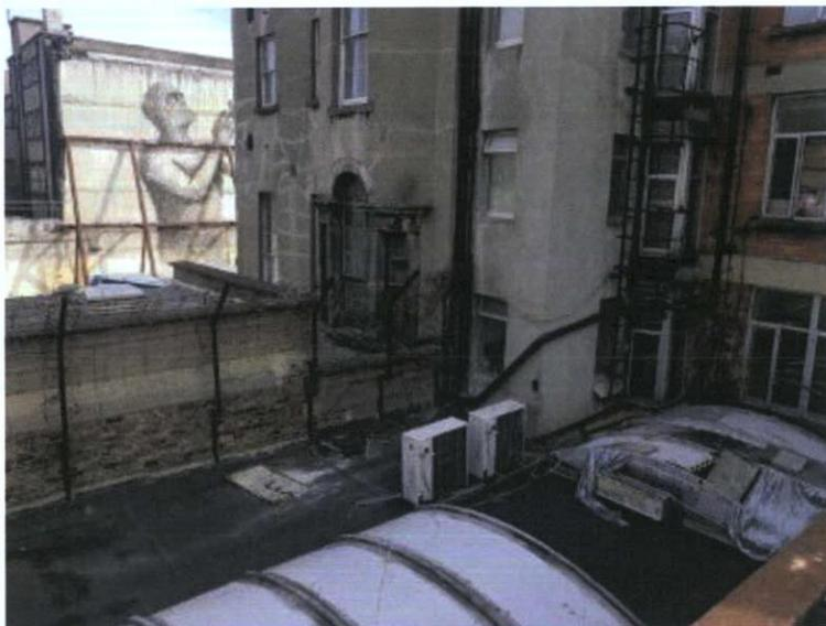
**Fig. 4** The eastern end of the boundary wall is attached to the rear of No.42. The flat roof above the rear extension of No.43 is dressed into the boundary wall.
